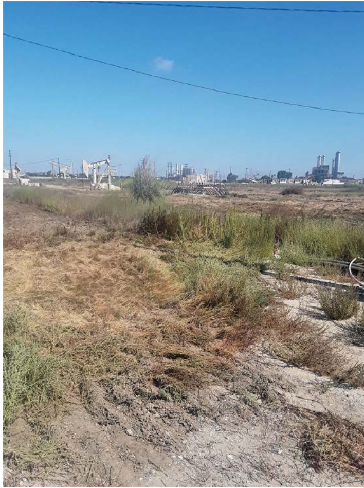
Photograph 2. Proposed Gas Plant ADI overview; view to the northwest.
